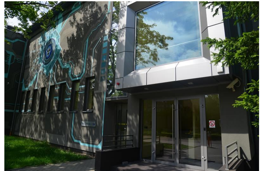
Świerk Computing Centre – main building
